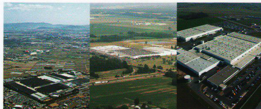
Takahama Plant - Japan
